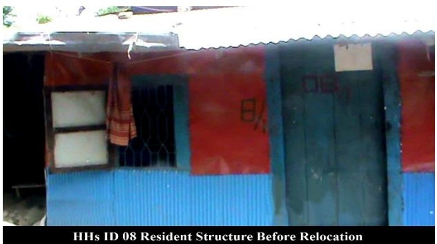
Photo 18: HH 08 before relocation in Polder-48
