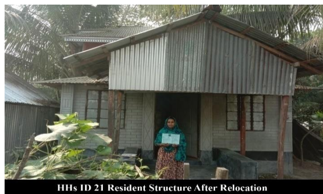
Photo 17: HH 21 After relocation in Polder-43/2C
