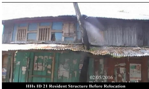
Photo 16: HH 21 before relocation in Polder-43/2C
