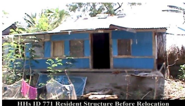
Photo 12: HH 771 before relocation in Polder-40/2
