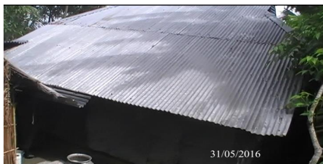
Photo 14: HH 377 before relocation in Polder-41/1
