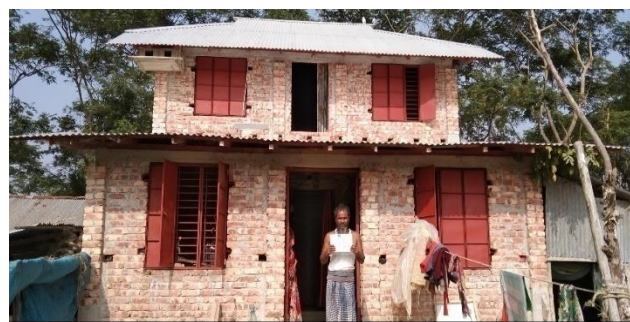
Photo 15: HH 377 After relocation in Polder-41/1
