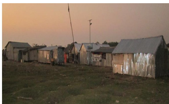
Photo 10: Khajura Group relocation of Polder-48
