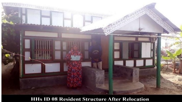
Photo 19: HH 08 after relocation in Polder-48
